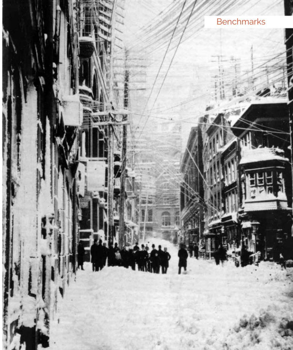
Ice- and snow-coated telegraph and telephone wires hang low on a New York City street. The storm exposed weaknesses in city infrastructure and prompted improvements, like the burial of electrical wires and the building of underground subway systems.
